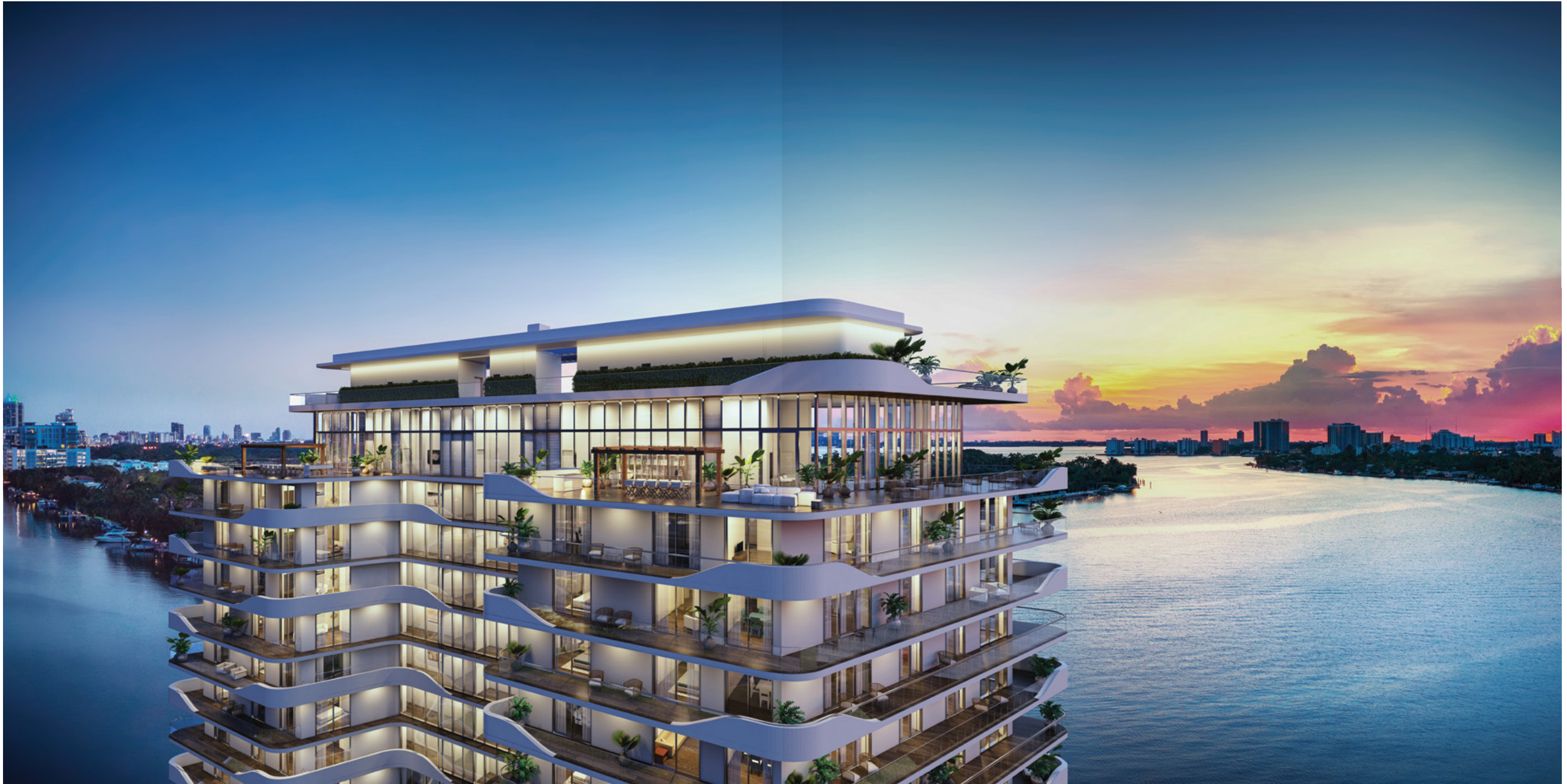
Two half-floor penthouses feature extra-deep, wrap-around terraces with east-to-west views of Biscayne Bay on one side and the Atlantic Ocean on the other. Equipped with electric outdoor grills, these privileged perches are the perfect place for alfresco dining.
